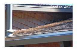
vegetative debris can readily accumulate at the intersections and so can burning embers. When the resulting fire is next to combustible siding or a dormer window it can cause the entire building to catch fire.
