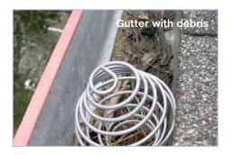
combustible siding. The metal gutter will remain attached to the fascia, and the ignited debris will burn out there, continuing to expose the edge of the roof. The most fire safe solution is to minimize the build-up of debris in the gutter.
